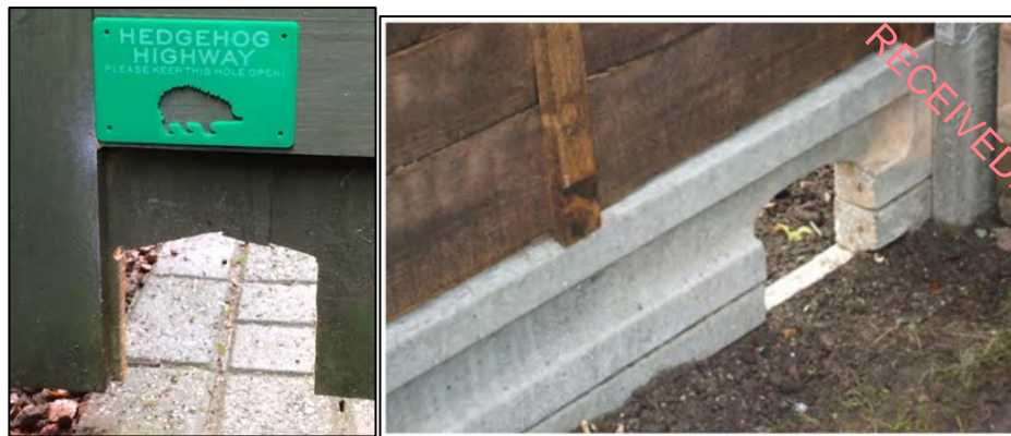
Figure 6.12: Examples of Hedgehog highways' that can maintain habitat connectivity for hedgehogs in residential developments
